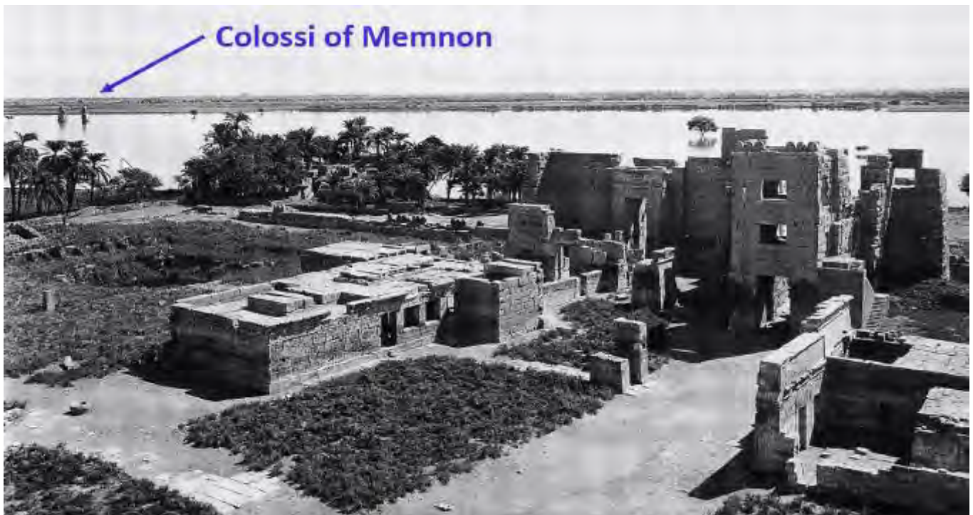
Inundation to the east of Medinet Habu, West Bank, Thebes
